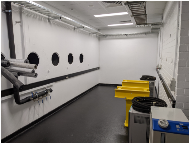
Figure 1: Beamline hall, a little over 8 m long
