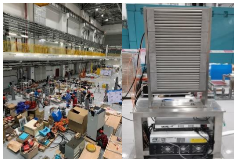
Bank assembly site
